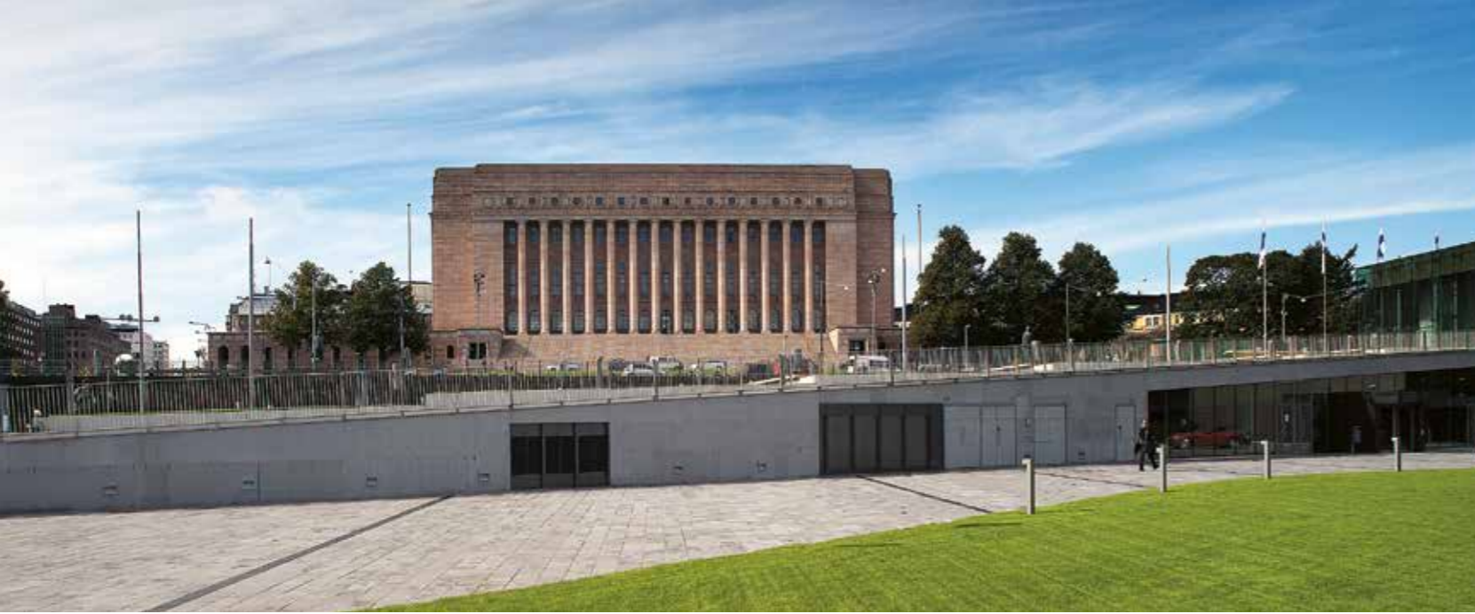
Parliament House was inaugurated in March 1931. The building, which is still today the foremost symbol for Finland's independence and democracy, was designed by architect Johan Sigfrid Sirén.
